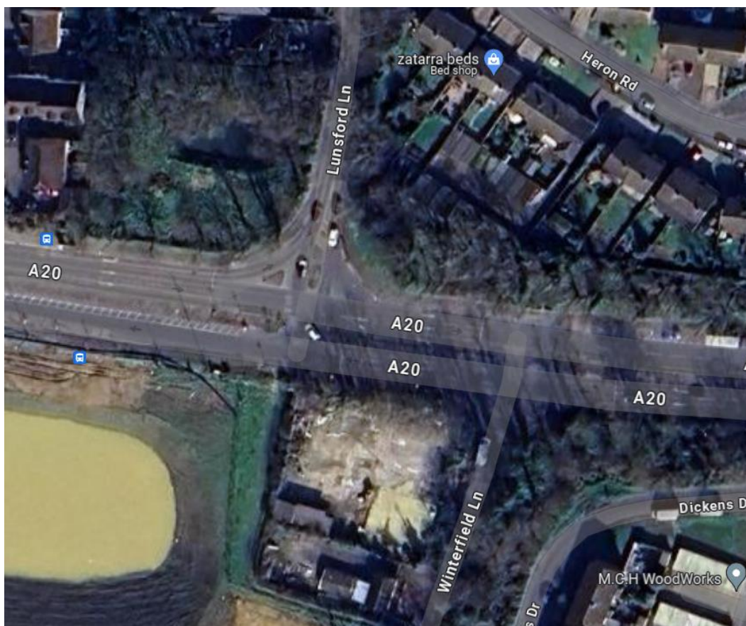
Figure 14-1: A20 / Winterfield Lane / Lunsford Lane Junction
