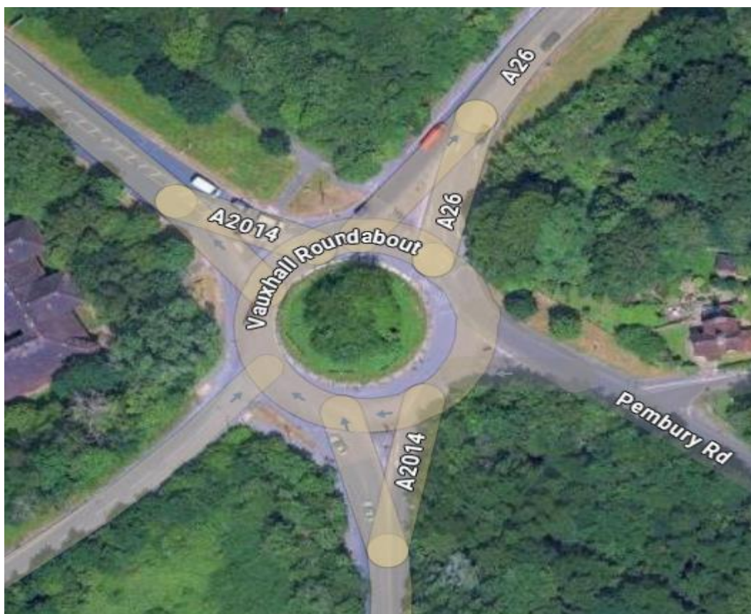
Figure 29-1: Vauxhall Roundabout Junction
