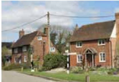
Buildings in Trottiscliffe
