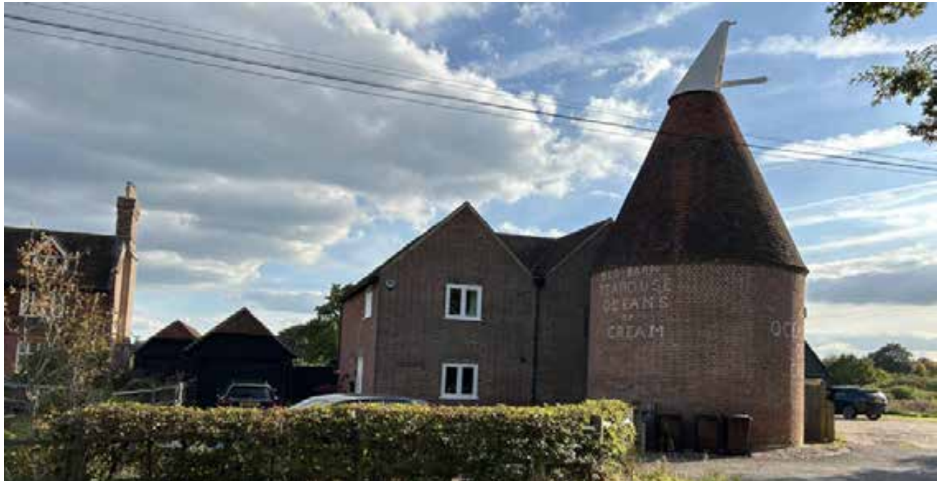
Oast House south of Stocks Green Road, formally the Old Barn Teahouse.
