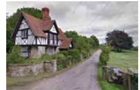
Gatehouse at Oxon Hoath Park
