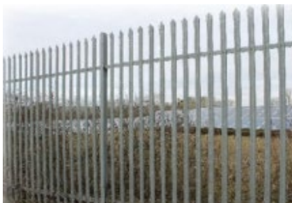
Solar farm enclosed by fencing
