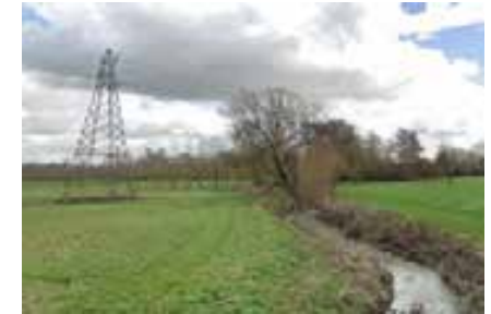
Pylons within fields
