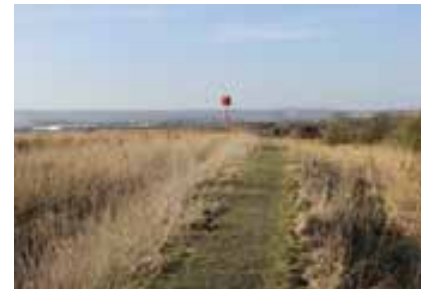
Footpath along river embankment crest
