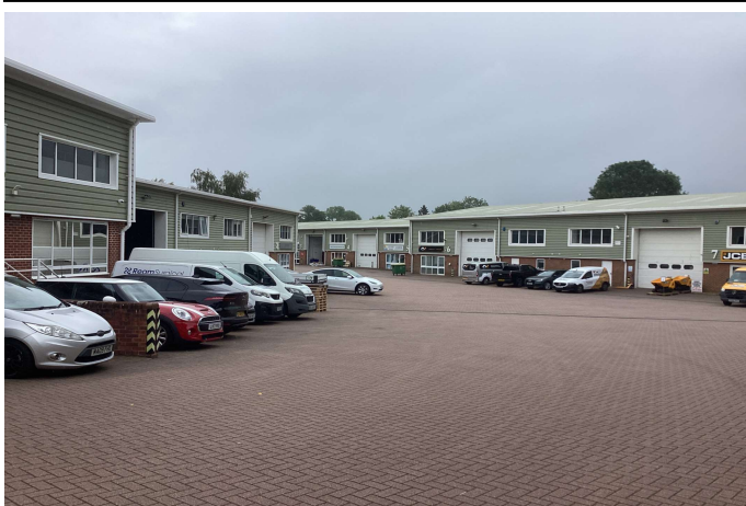
Looking south-east from within the sub-area, showing office and light industrial buildings and associated car parking.
