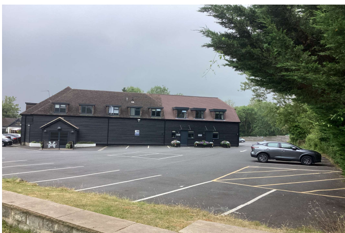
Looking south-east from an eastern point on the northern boundary, showing a pub and associated car parking.
