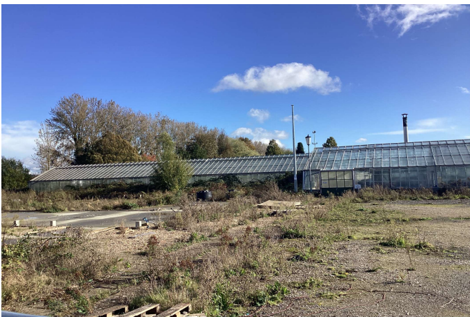
Looking east from within the western part of the sub-area, showing disused agricultural greenhouses and an overgrown area of hard standing.
