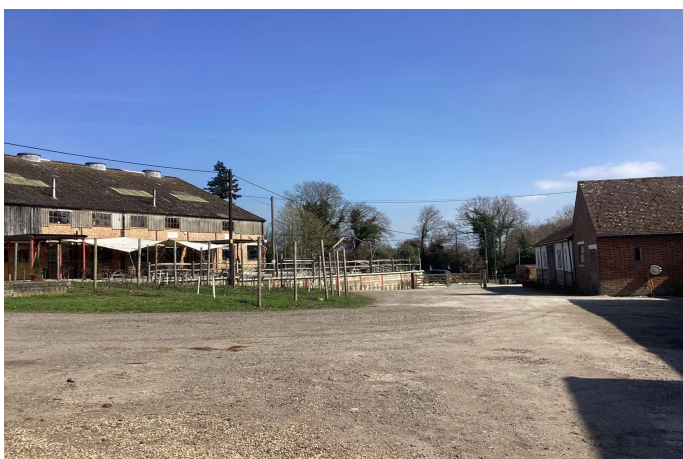
Looking east from the south-west corner of the sub-area, showing an area of hardstanding and light industrial and commercial premises associated with a winery.
