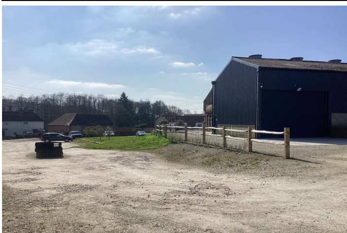
Looking south from the north-east corner of the sub-area, showing commercial and light industrial buildings associated with a winery, and an area of hardstanding.
