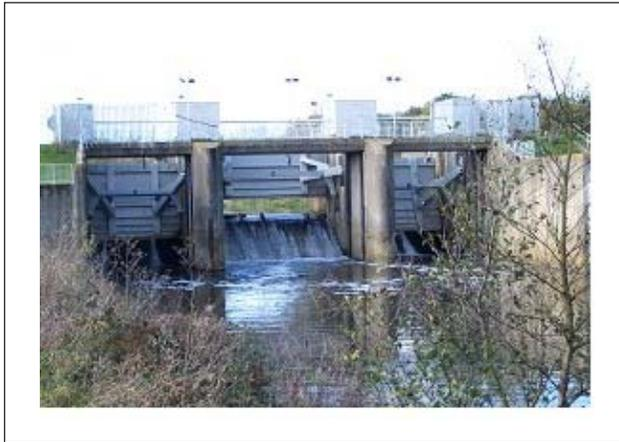
The storage area behind the Leigh Barrier is 278 hectares (686 acres) (that is about 255 football pitches), and when the land is flooded it can hold 5,580 million litres of water (1,230 million gallons). Before the barrier was constructed Tonbridge would regularly flood – the last serious floods being in 1968. See [www.environment-agency.gov.uk](http://www.environment-agency.gov.uk) for more information about the barrier.
