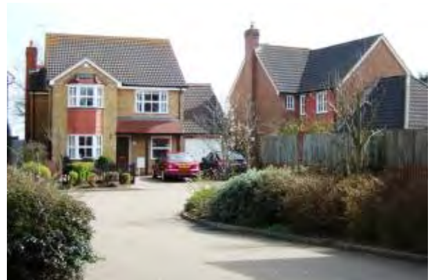
Spa Close is a recent development of detached houses set around a shared access. Two pairs of houses flank the entrance facing onto the Maidstone Road behind landscaped front gardens enclosed by brick walls and shrubs. The detached houses are constructed of brown and pale yellow brick and incorporate details including contrasting brickwork, tiled pitched roofed porches, tile hung two storey bay windows and decorative ridge tiles. The character is enhanced by shrub planting.
