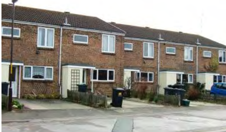
The houses in The Paddock are constructed of brown/buff or red brick. The terraced houses are of consistent design with shallow pitched brown roofs and flat roofed, rendered front porches uniformly painted cream. They have vertical and horizontal windows and open frontages with picket fences on the side boundaries. The uniform design and colour scheme gives the development a strong identity.
