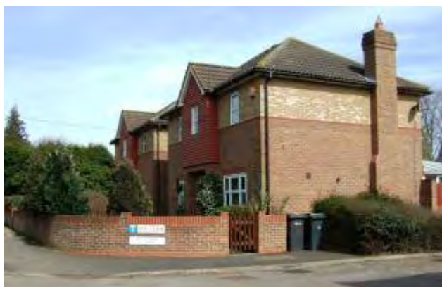
Spa Close is a recent development of detached houses set around a shared access. Two pairs of houses flank the entrance facing onto the Maidstone Road behind landscaped front gardens enclosed by brick walls and shrubs. The detached houses are constructed of brown and pale yellow brick and incorporate details including contrasting brickwork, tiled pitched roofed porches, tile hung two storey bay windows and decorative ridge tiles. The character is enhanced by shrub planting.
