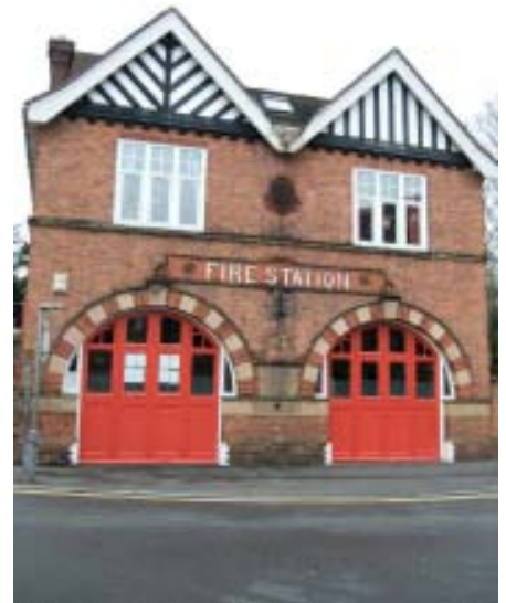
Former Fire Station – a new focus for public realm improvements
